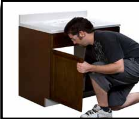
Step 2 ADA VANITY: Carefully remove doors and set aside for later use
