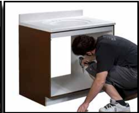
Step 5: Remove floor screws (4)
