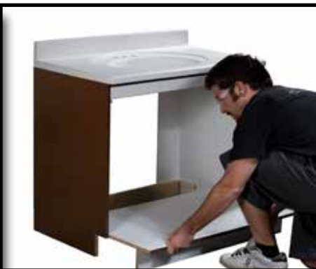
Step 6: Slide floor board out and set aside for later use
