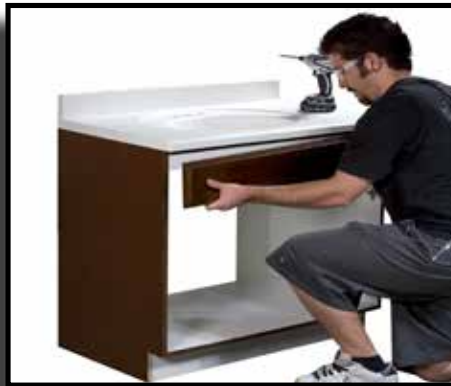
Step 4: Unscrew header from bracket with normal Phillips Head screwdriver
